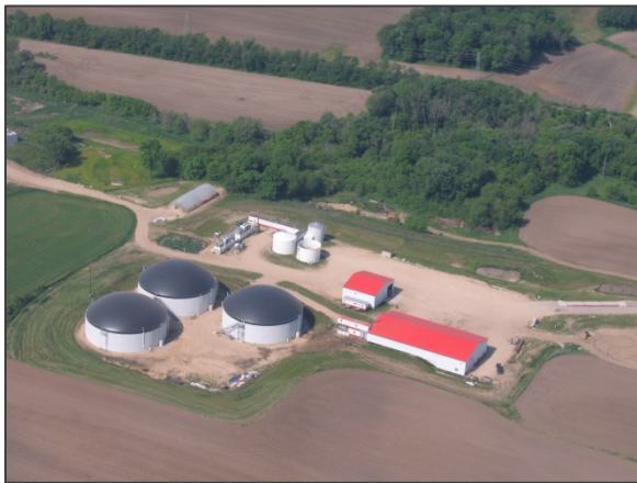
Cow Power manure digester, Waunakee
